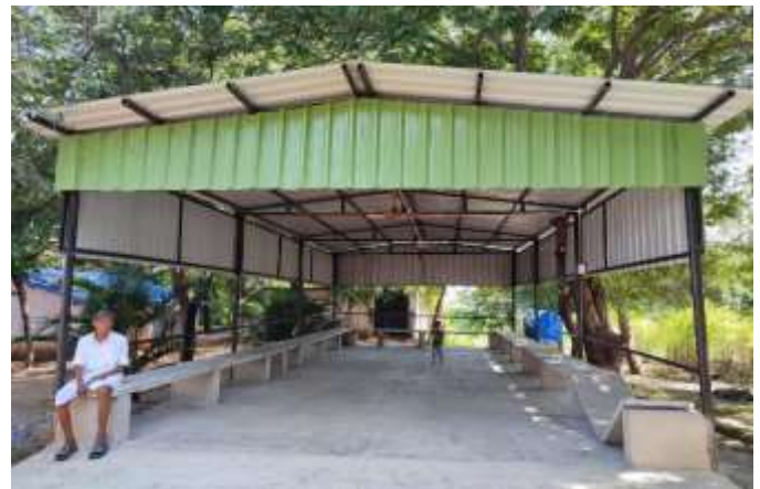
The new spacious shelter complete – October 2022
